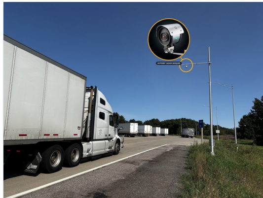
Typical field installation. A Kingfisher sensor pole-mounted at a facility entrance with its roadside control cabinet.
